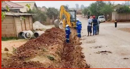
STORMWATER DRAINAGE CONSTRUCTION
